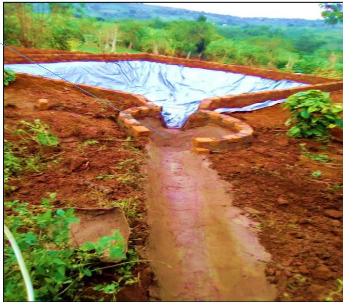
A rain runoff pond with a small soil collecting pond before the main water pond (source: www.med6agrotech.com )
