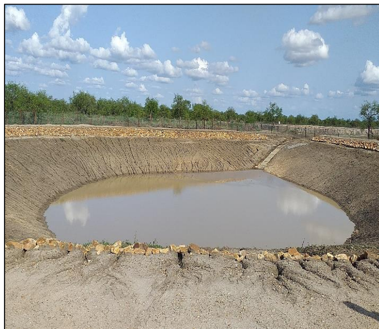
Ground surface runoff harvesting, into a valley tank (source: www.med6agrotech.com )
