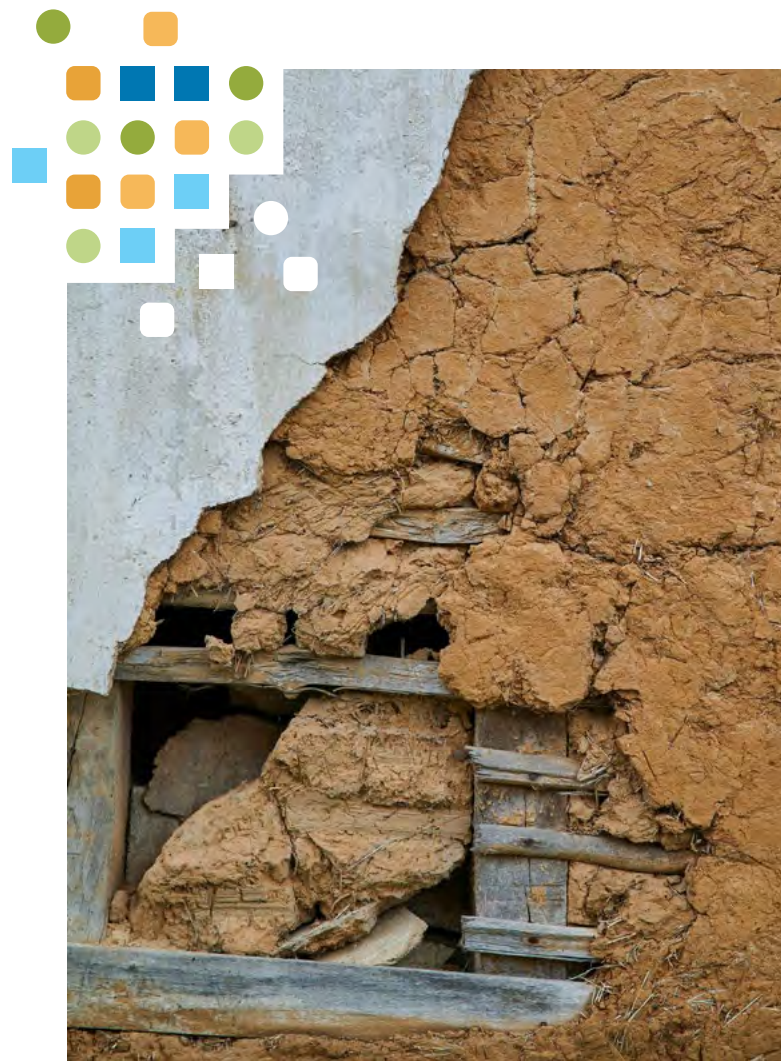
A close-up of a layered wall of a building made of natural and reusable materials such as clay Unsplash/Johnny Goerend
