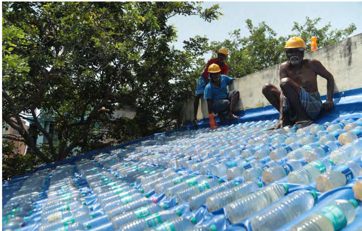
Building a low-cost roof cooling-system made of PET bottles in Chennai, Tamil Nadu, India | GIZ
