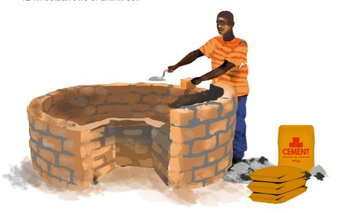
Most of the materials Amake Willie used to construct her pan-brick KHG are locally available. She also advised us to avoid plastering the inside of the KHG wall as this affects porosity resulting into waterlogging and poor plant growth. As a family, we will mould and burn enough pan bricks and sale some chickens to raise money for buying cement and construct a strong KHG which can last longer.
