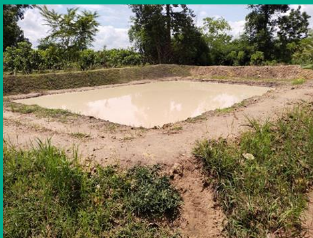
Muddy pond because of dyke erosion
