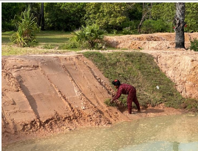
Figure 17: Planting grass on pond dykes for stabilization Photo credit: Theo Ebberts/GFA, SAFR project
