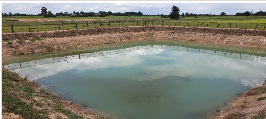
Figure 24: Dug out pond with "flat" and "stepped" slopes to protect against erosion
