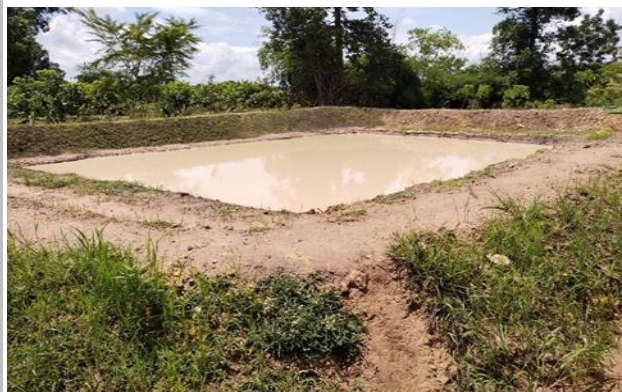
Figure 64: Muddy pond due to pond wall erosion
