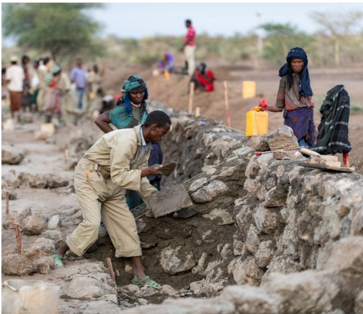
Training programme for local communities in masonry work for the construction of WSW in Ethiopia's lowlands (Afar).
