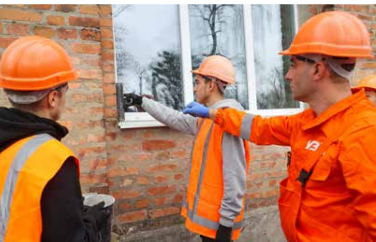
Build back better: Vocational school students in Kharkiv learn how to install energy-efficient windows in the war-damaged school building.
