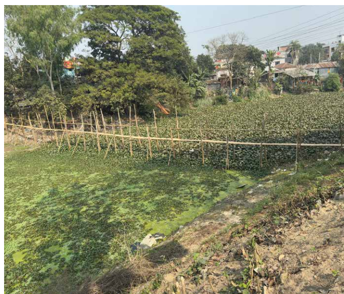
Community made bamboo bridge constructed over canal
