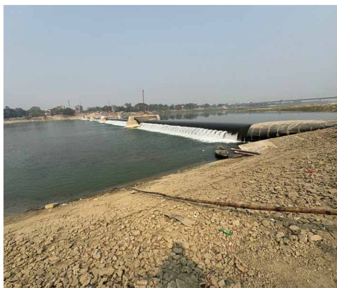
Rubber dam to reserve water for household supply and irrigation during dry seasons
