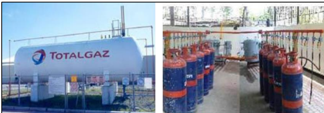
Figure 33: Central tank (left) cascade system (right)
