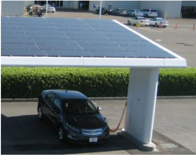
Figure 31: BIPV charging station 27
