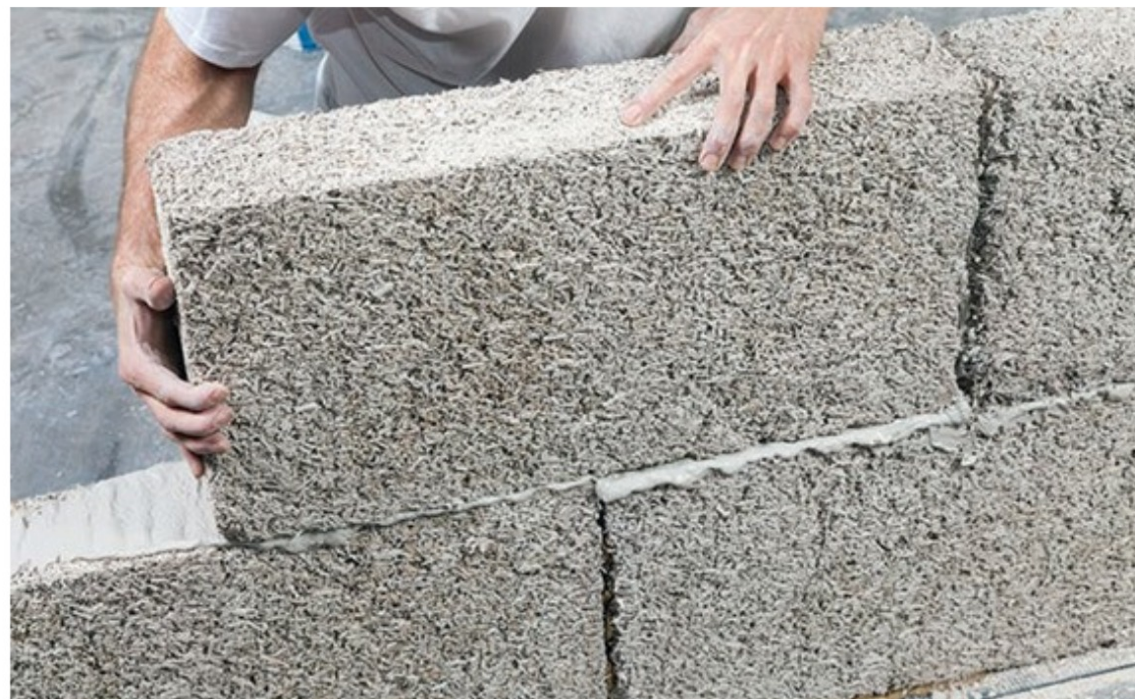
Hempcrete blocks made from hemp shives and lime. They offer high acoustic and thermal comfort, as well as high fire resistance.
