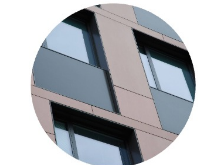
HICEM / Fibre Cement Board 7-9 kg CO2e / m2
