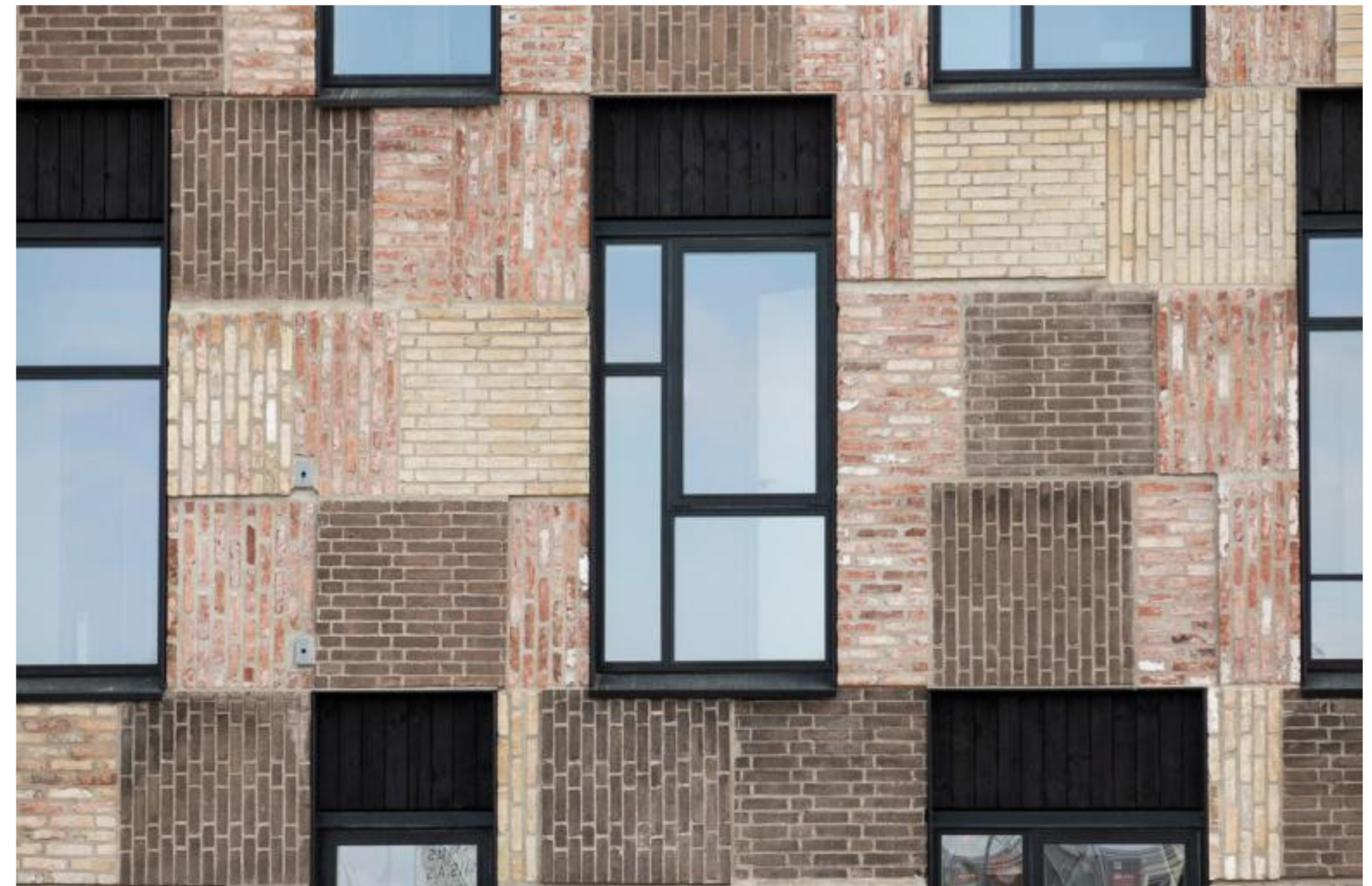
The brick modules at the Resource Rows in Copenhagen were cut out of old buildings at the Carlsberg Brewery. Lendager Group, 2019, Photo © Lendager
