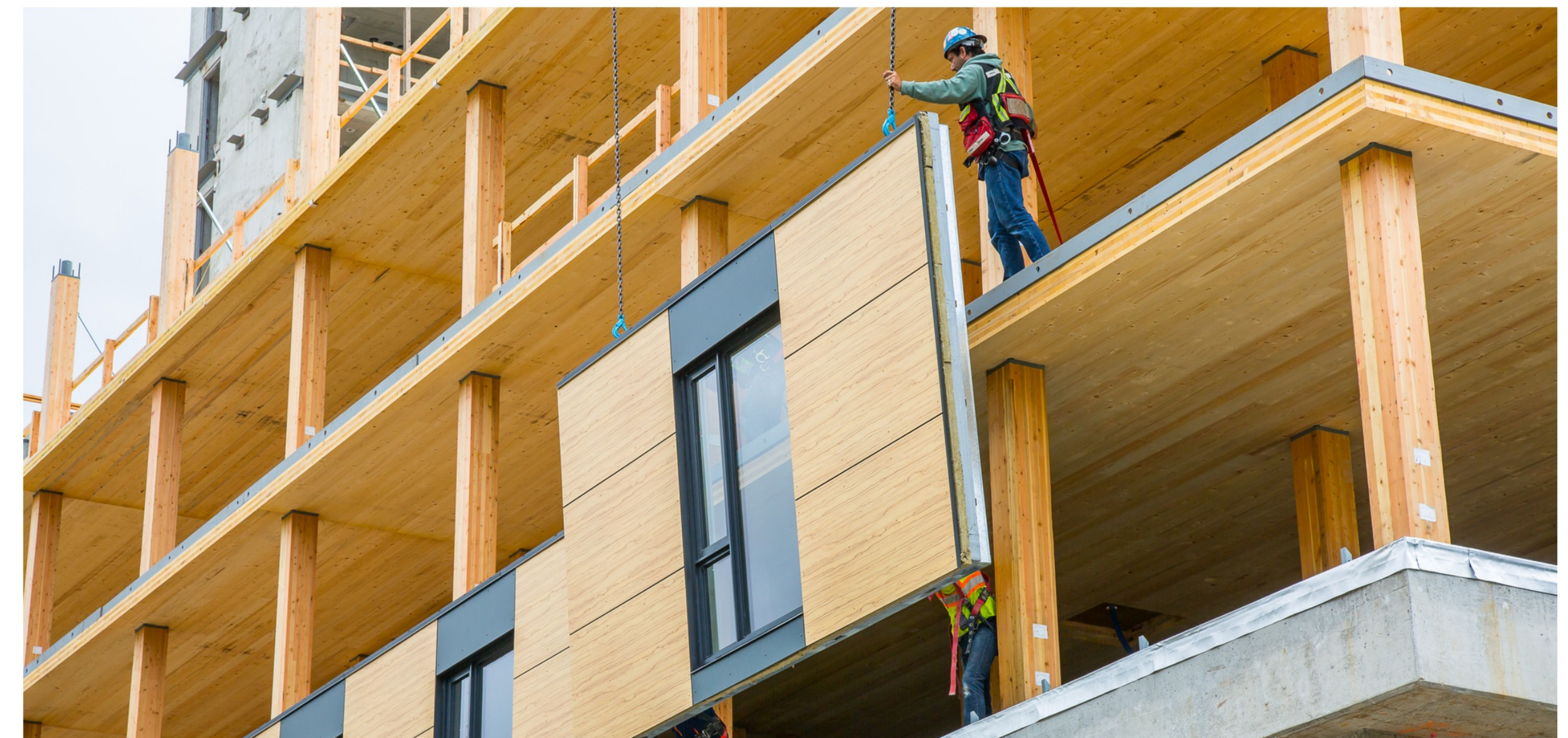
Tallwood House is an 18-storey mass timber hybrid student residence at the UBC Vancouver campus. © Living Labs UBC, https://livinglabs.ubc.ca/projects/brock-commons-tallwood-house
