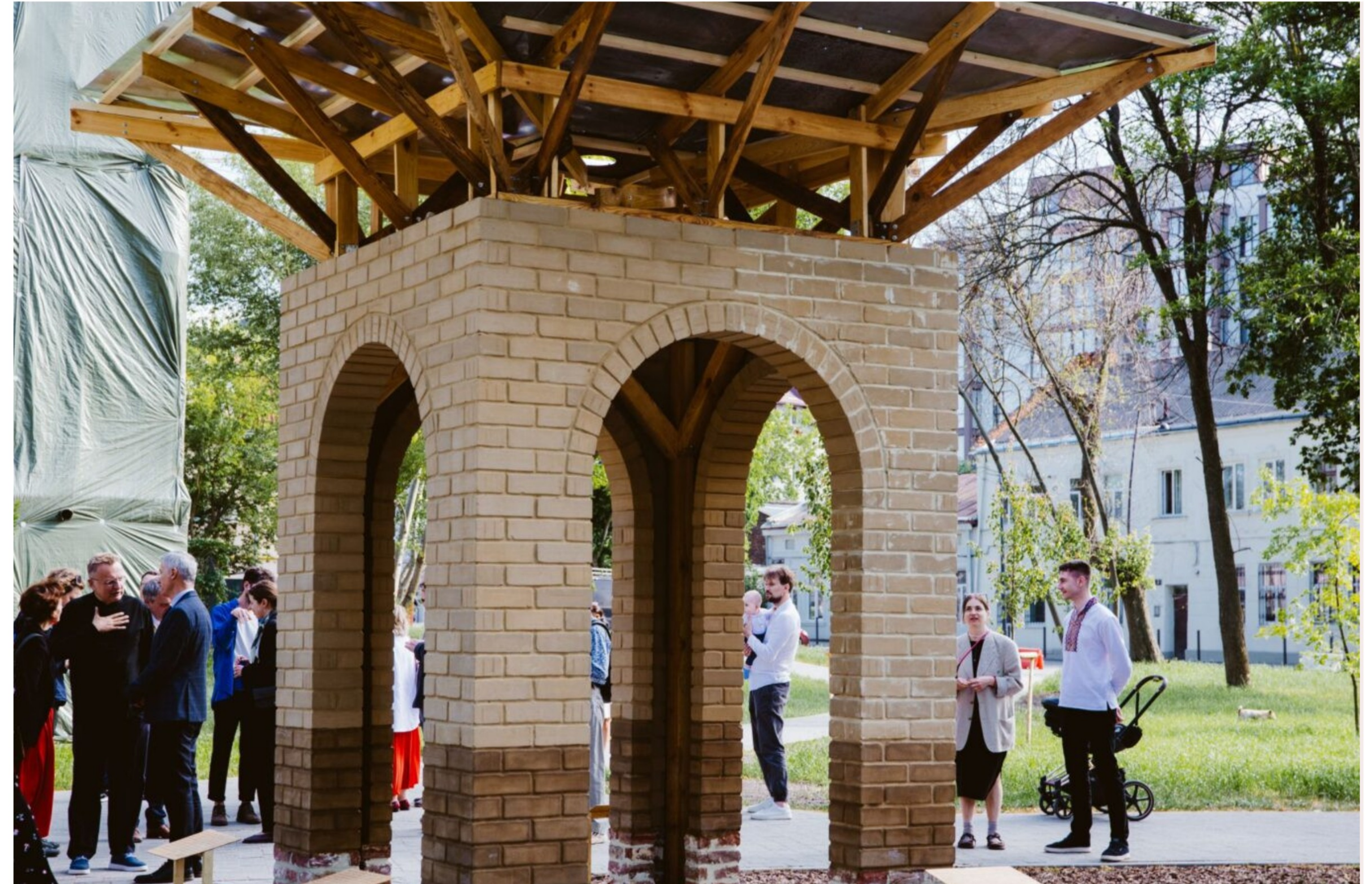
Earth Pavilion and Reclaimed Materials in Lviv. Project by Anna Pommazana & Mykhailo Shevchenko. Grunt Experimental Fellowship with Bauhaus Earth. Photo © Zlatoslava Kryshchak
